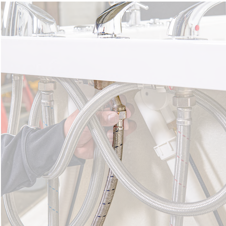
Tighten the other end of the supply hose on the available spot underneath the center valve (diverter) of the Ella 5pc faucet
