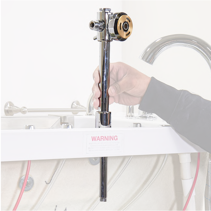
Place and secure the shower column to the deck of the walk-in tub
